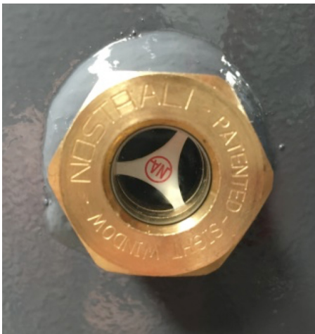
✗ Completely Empty Tank
