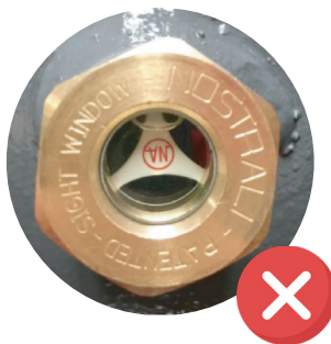
Completely Full Tank
