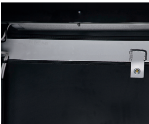
Optimised Cooling System for 122°F High Ambient Temperature
