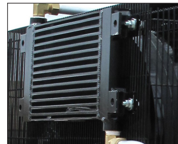
Air cooled after cooler Platinum unit
