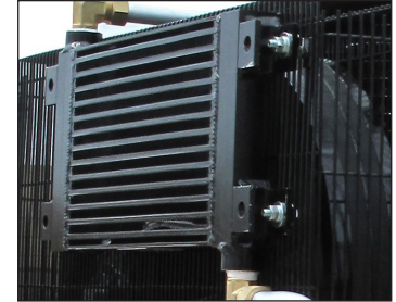
Air cooled after cooler Platinum unit
